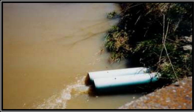
Photo of tile outlets along an open ditch in Howard County. Outlets receive water from several tiles draining a field.
